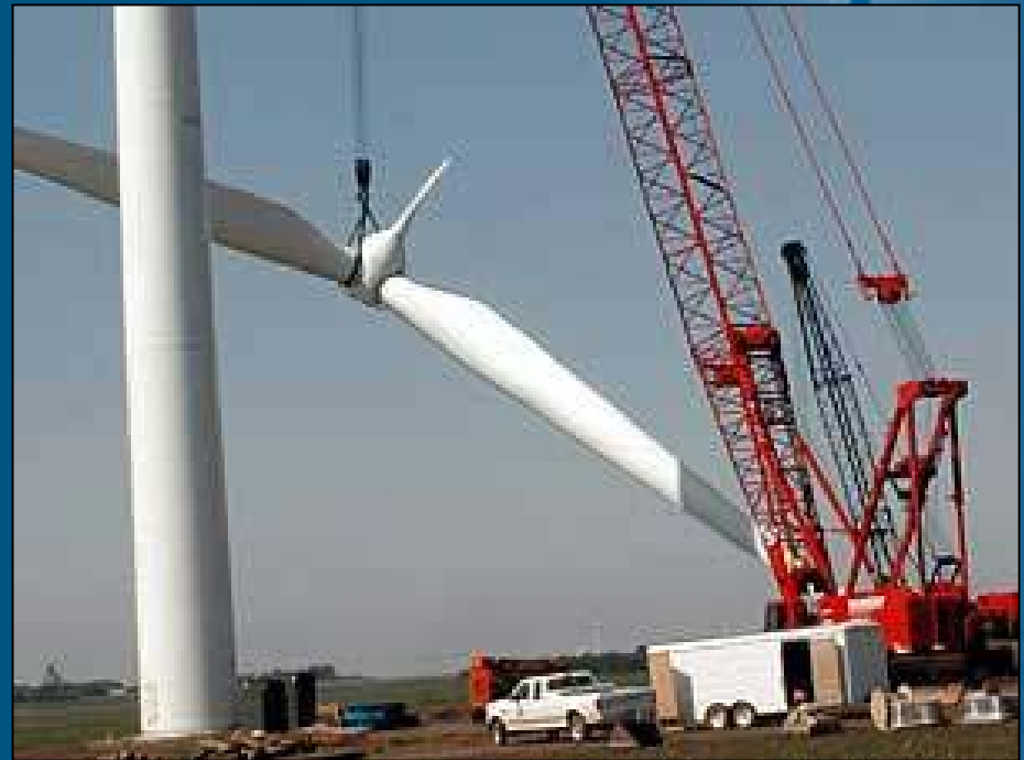
Fey family wind turbine under construction. Photo by Mark Steil/MN Public Radio
